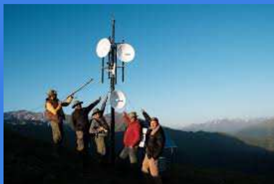
Figure 4 : Station de base
